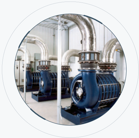
A bank of three Spencer Power Mizer blowers operating in parallel for wastewater aeration at a large wastewater treatment plant.
