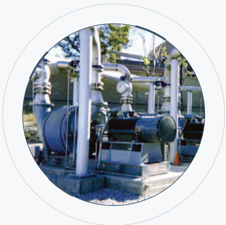
Three Spencer Power Mizer Series 7000 blowers supplied with Heresite® coated internal parts are installed at a California municipal landfill gas facility for handling extremely corrosive and combustible gases.
